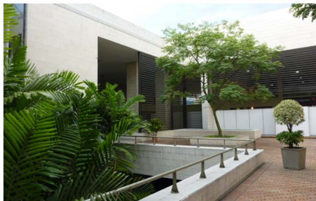
Conference Center in Cali, Colombia. The center has been built in conformity with "green building" criteria. Source: Thierry Buchs, SECO
